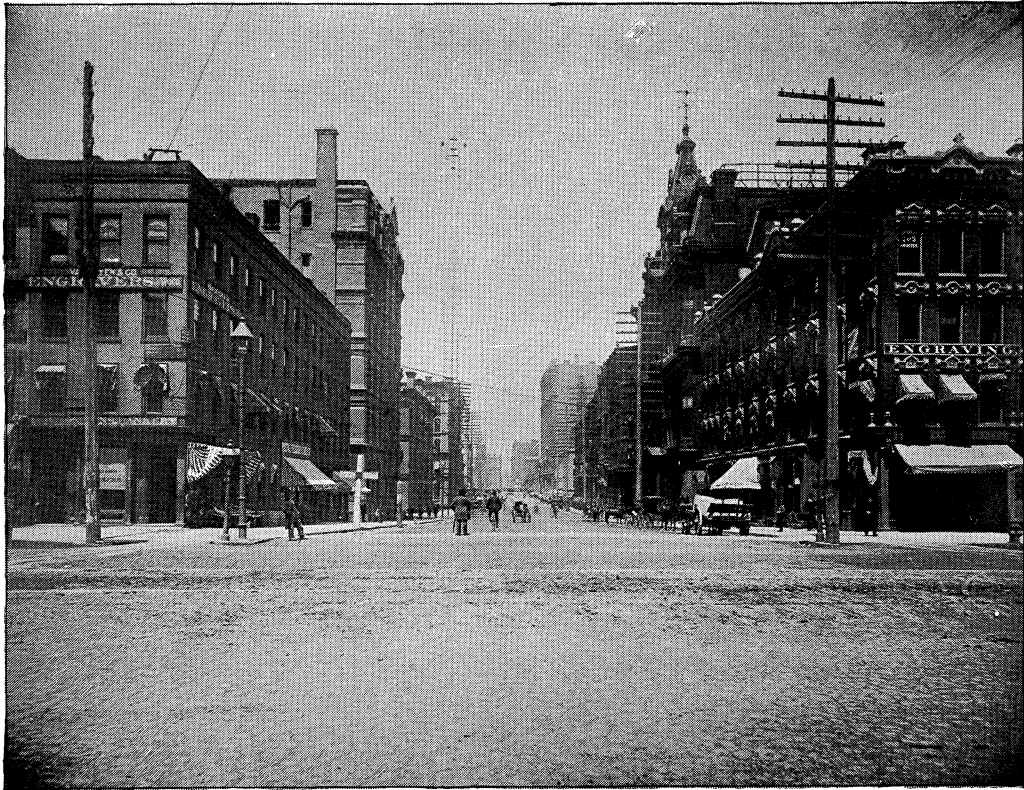
STREET VIEW, LOOKING NORTH ON GRISWOLD STREET, FROM JEFFERSON AVENUE.
